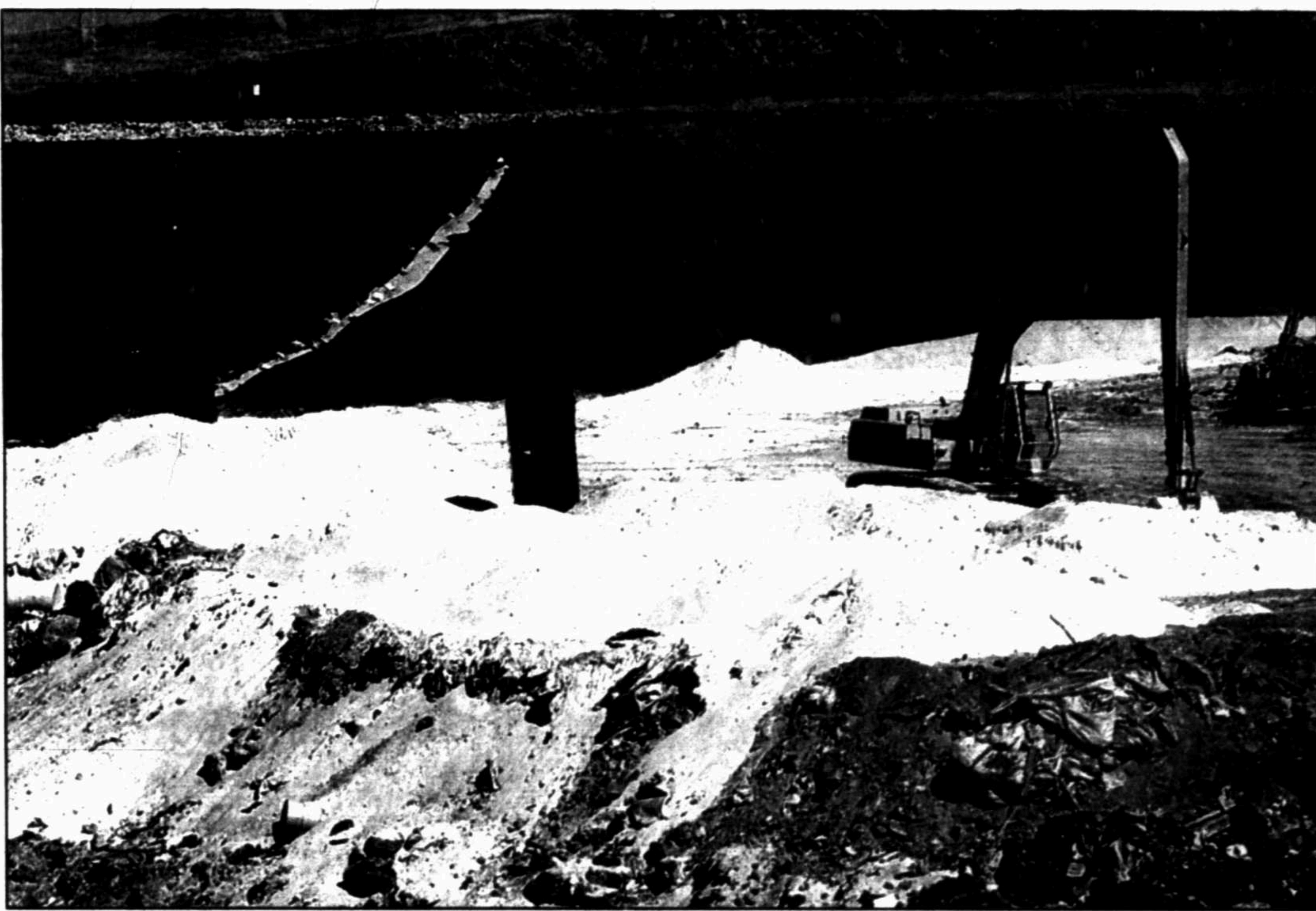
ABOVE: A Waste Control Specialists landfill is designed to contain all waste underground. The long, black drainage pipes pump rainwater out of the hole and into a storage tank. The light-colored material in the hole is sand used to cover the waste. BELOW: Tooele County's (Utah) multi-sport complex, is under construction, to attract sports events. The complex will include a football stadium, rodeo arena, small racetrack, swimming pool, softball baseball and soccer fields and an activity building.
