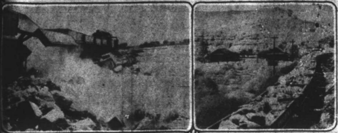
Above are two views of the "first" defenses in the Imperial Valley against the Colorado river. At the left a train is shown crossing a bridge over the Andrus levee; at the right a rock train is shown winding across the desert to a threatened point. The map shows the location of the upper point, with levees, canal and river indicated. The Imperial Valley lies near El Centro, in the upper right hand corner of the map.
