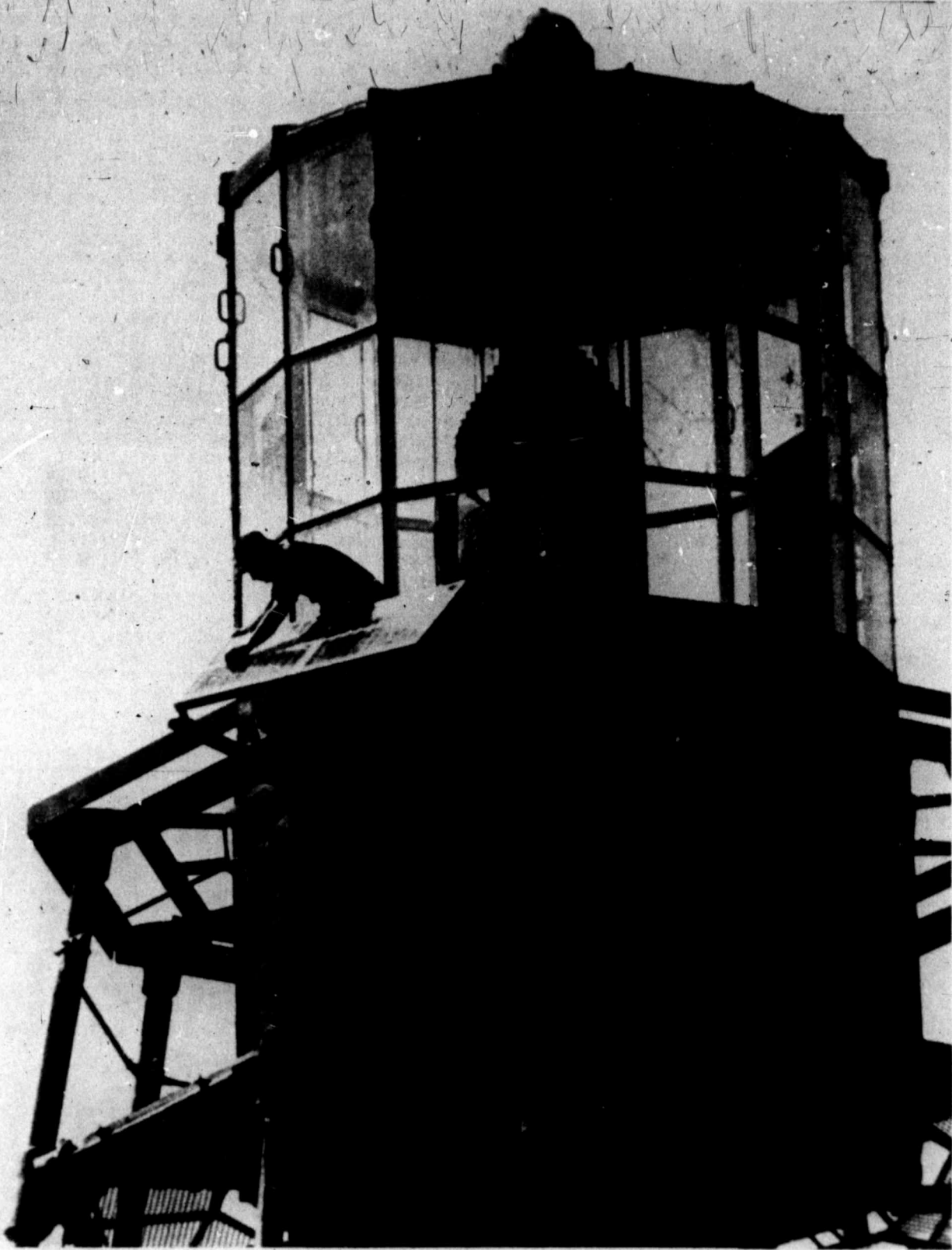
GEORGE MATRIGALI WORKS on the solar panel that powers the 110-foot Caresfort Reef lighthouse
