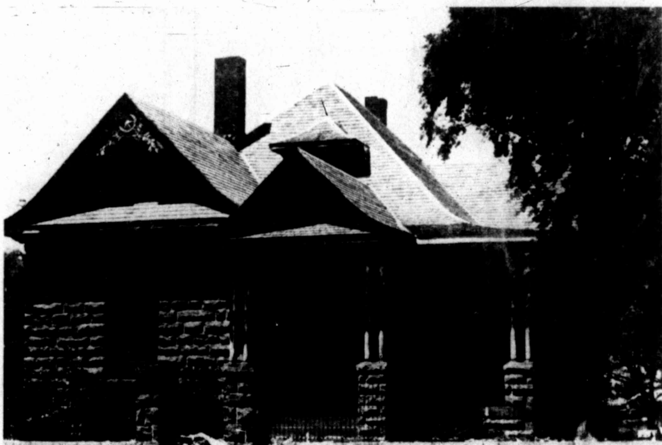
Restoration of Big Spring's Potton House is under way.
