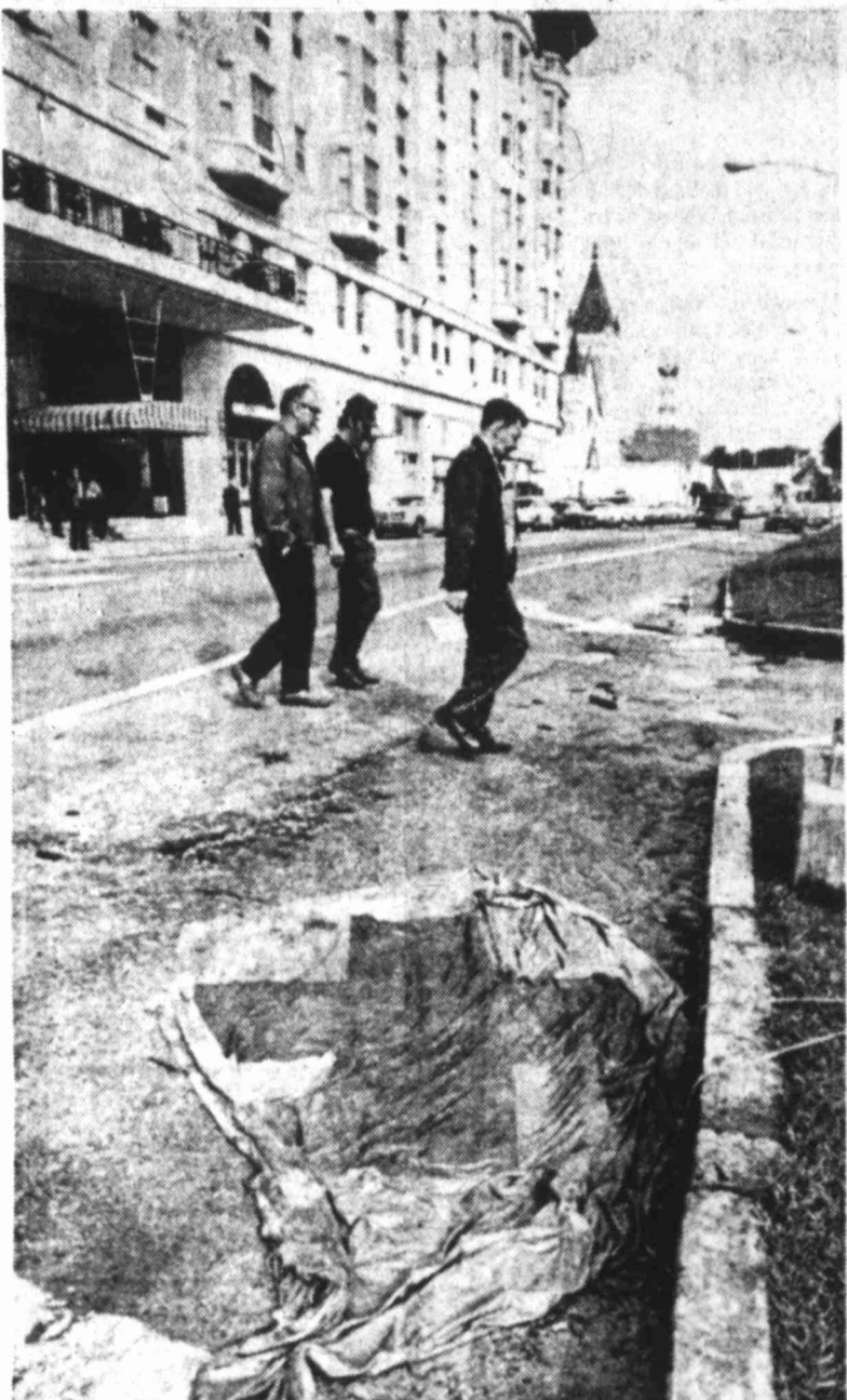
DOWNTOWN SURVEYED AFTER FLOODING — A muddy Red Cross emergency flag lies in the gutter of a main street in downtown Pensacola, Fla. Sunday as residents survey the damage after 14 inches of rain fell there Saturday. (AP Laserphoto)
