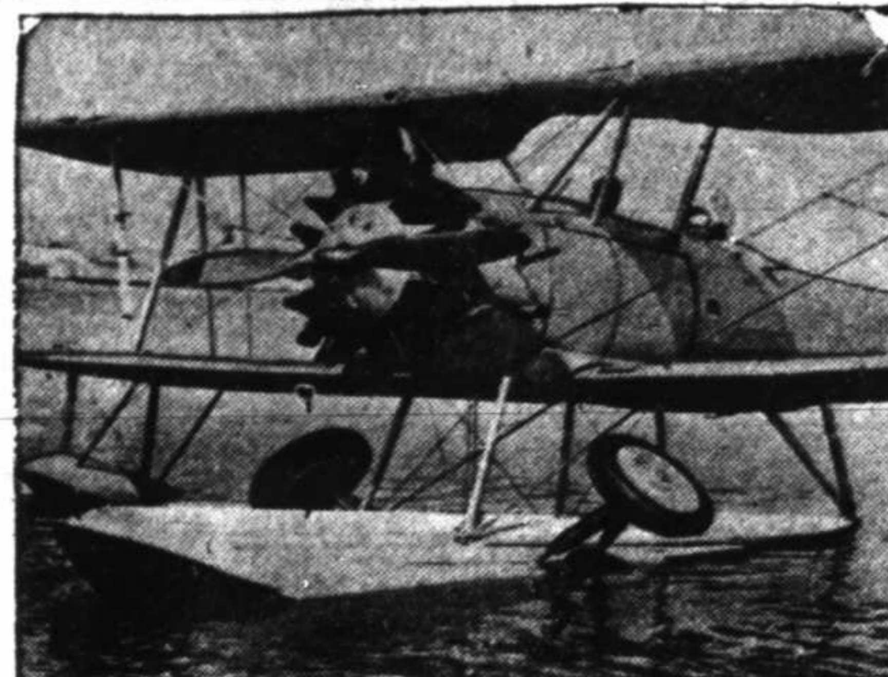
CLOSEUP OF WASP VAUGHT AMPHIBIAN SHOWING WHEELS IN FLYING POSITION
