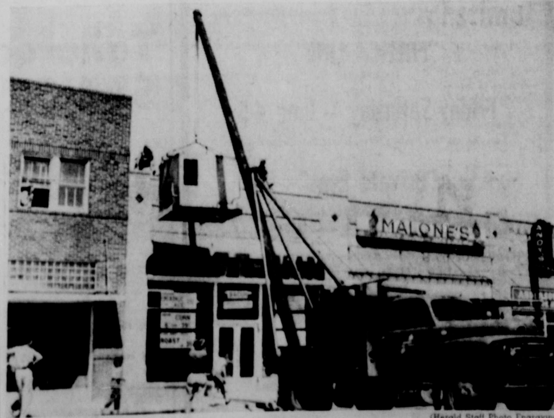
TICKLISH JOB —A lot of sidewalk superintendents gave advice as workmen of the Community Public Service Co. moved this huge air conditioner from the roof of the former Kelley Drug to the roof of the Burk Corner Drug, a few doors south. All this moving took place last Friday.
