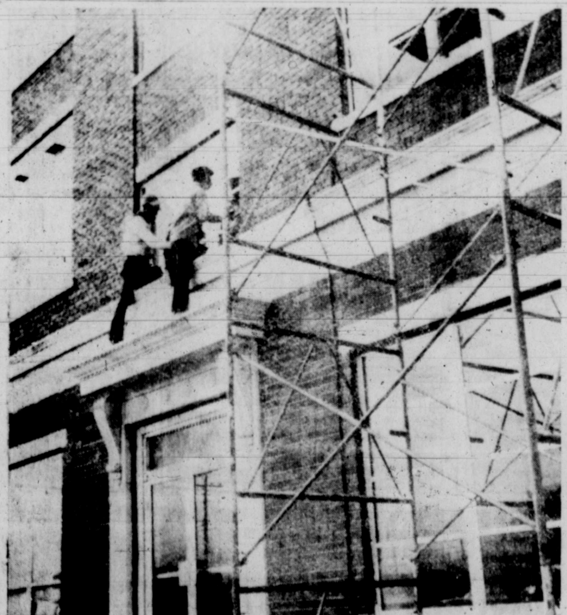
Finishing Touches On The Courthouse
