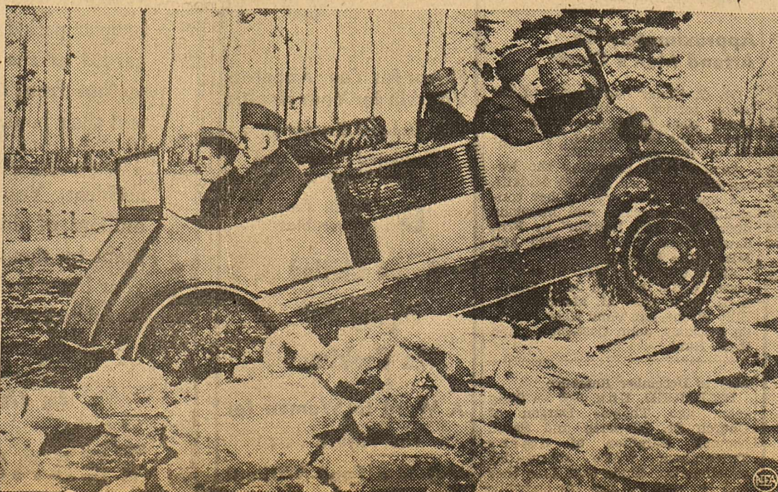
Holland finds her flood defenses still in working order as army amphibian car, bogged down after breaking through thin ice during test maneuvers, is unable to regain the frozen surface and advance.
