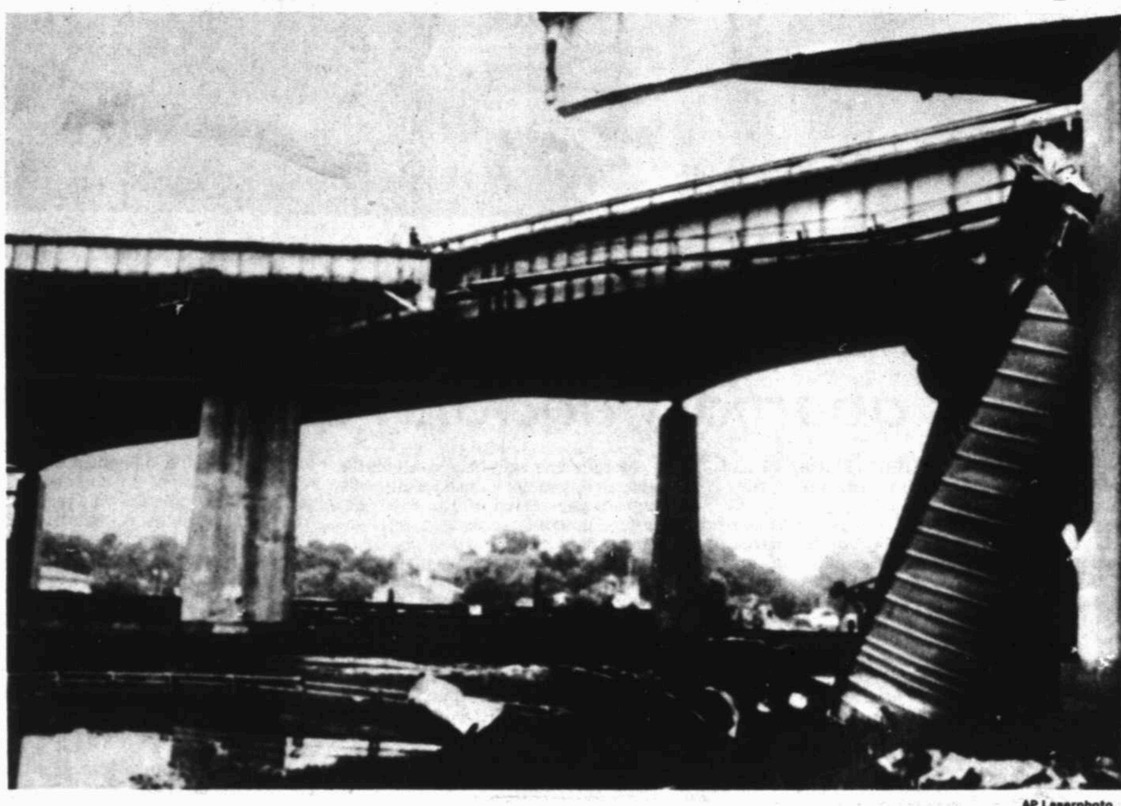
A trailer truck leans against an abutment of the Interstate Highway 95 bridge over the Mianus River near Greenwich, Conn. The bridge collapsed early today, killing three persons and injuring at least three.
