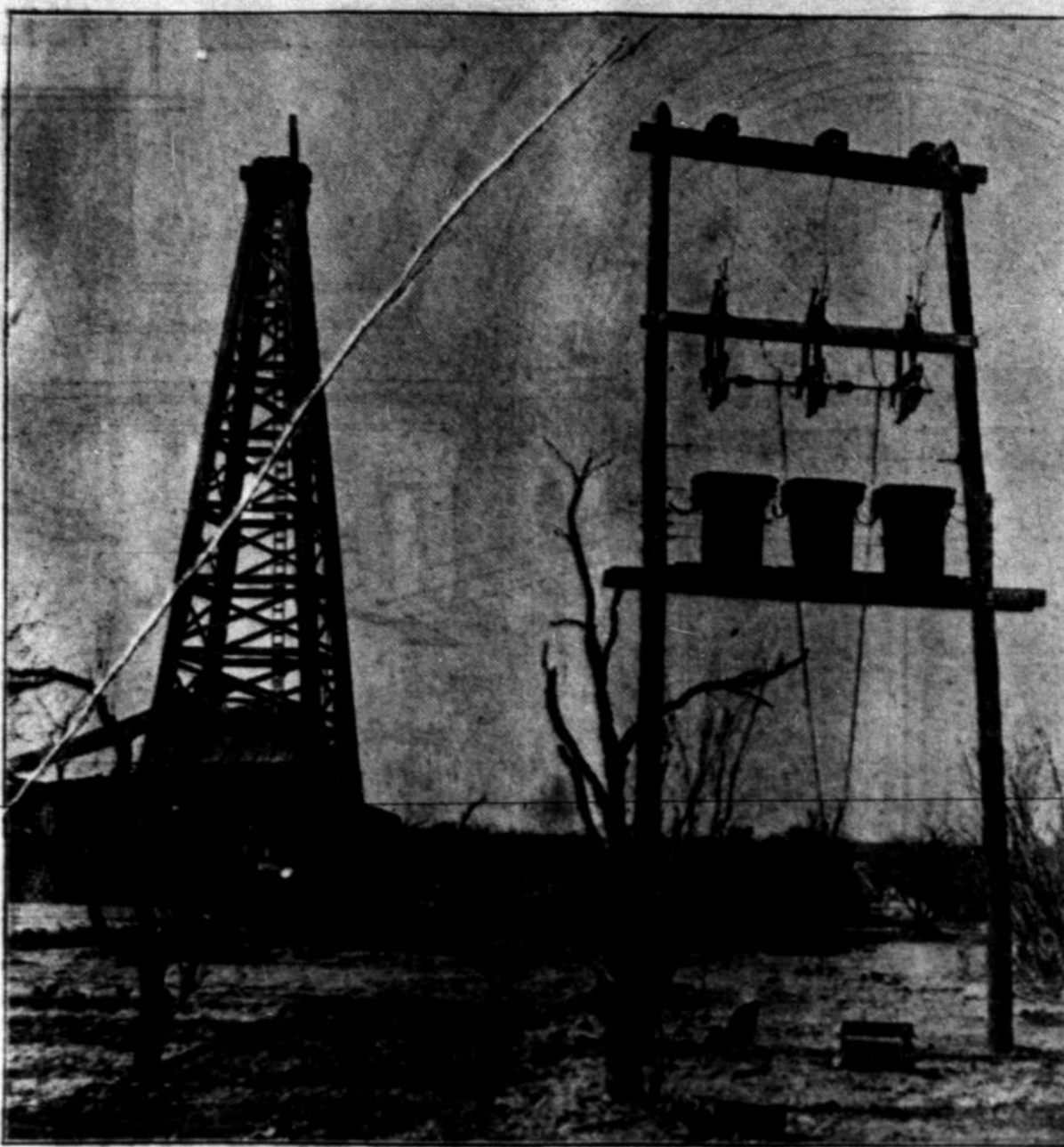
Contrast with a vengeance! The old-fashioned wooden derrick with its gas engine, and beside it the electric high line and "step down" line carrying power to many oil wells.
