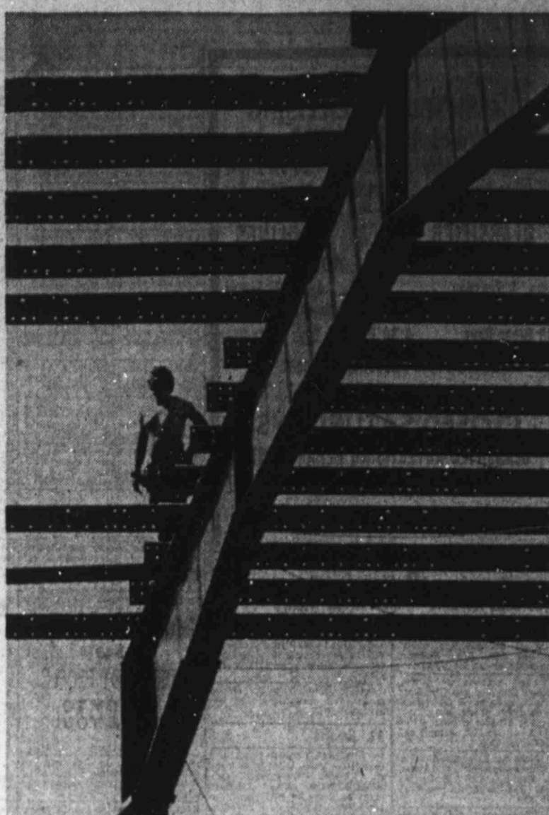
FAIR GIRDS UP — A workman waits atop steel girders etched darkly against the bright sky. The work is for a 25,000-square-foot addition to the Auto Exhibit Hall at the State Fair of Oklahoma at Oklahoma City. (AP Laserphoto)
