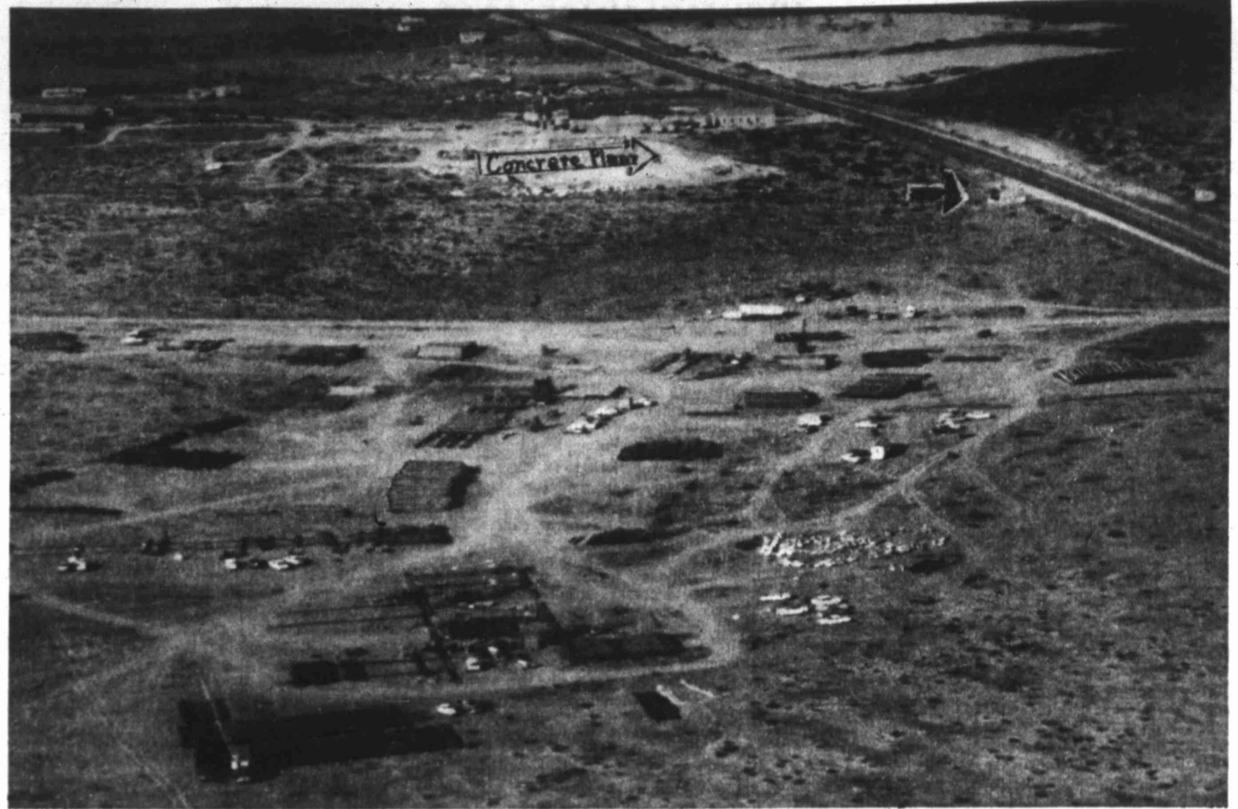
Scene Of Pipeline Reconditioning
