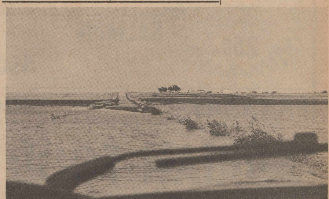
SLOW -- On second thought STOP! Recent rains presented area drivers with certain difficulties. Sometimes, and this was one of the times, inundated roads required drivers to GO AROUND.
