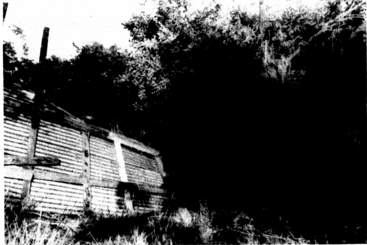
An isolated wind storm apparently scattered parts of a structure from the Boyd Street property of Manuel and Vicky Lopez in Colorado City along a path a block long on Monday afternoon, although no other reports of wind damage were reported in the area. Here portions of the structure's roof are shown at the edge of McKinney Street, a block behind the property.
