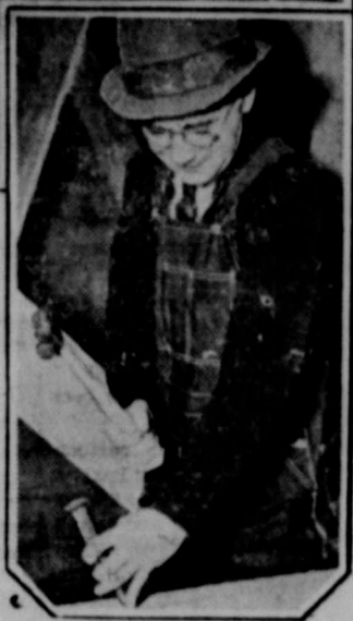
Reverend Brdlik is pictured at work on the new Brookfield, Ill., Baptist Church, shown under construction.
