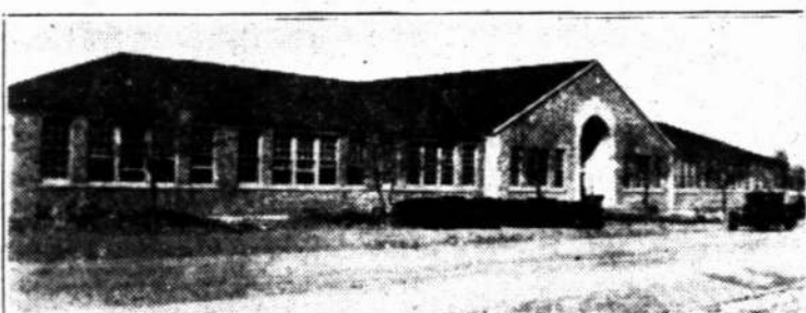
Rapidly nearing completion is the new $75,000 Grammar School building in Seminole pictured above. This structure will help house the more than four hundred students who are enrolled in the Seminole schools. WPA funds were a great help in the construction of this modern new structure. The exterior is finished in a light cream colored face brick. It will not only be a credit to Seminole, when completed, but would do justice to a town many times the size of the Gaines County Capitol.
