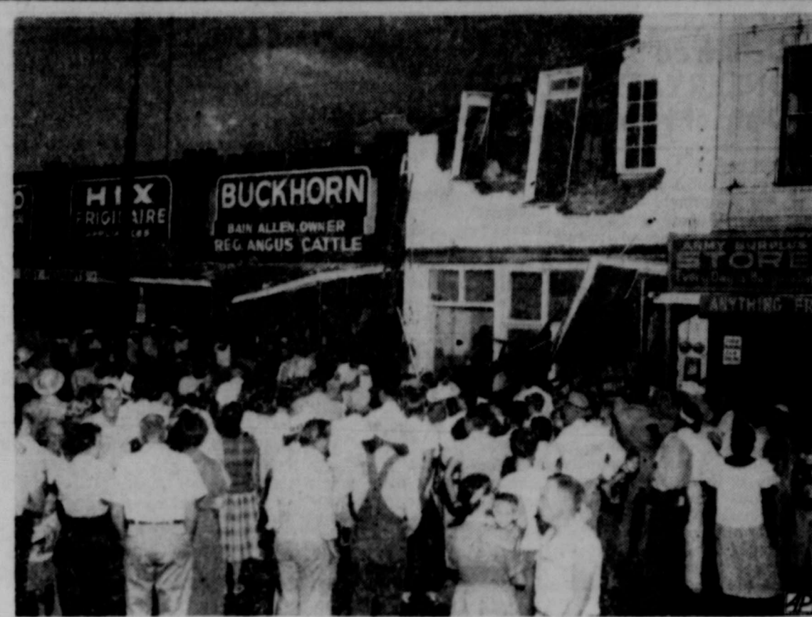
TWO DEAD IN BUILDING COLLAPSE—A blast of wind from a sudden thunderstorm toppled this two story building in Gatesville, Texas and debris fell onto the building next door, killing two men and in juring a woman. The buildings housed a cafe and domino parlor, a barber shop and another cafe. (AP)
