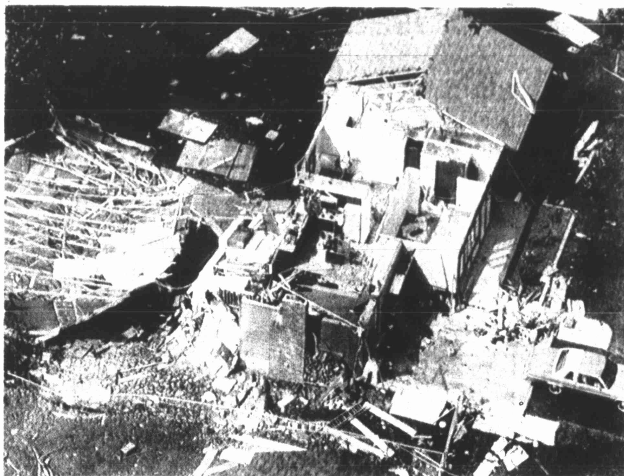
Little remains of what used to be a home in Maple Grove, Minn., which was devastated by a tornado packing winds of 160 miles per hour Thursday night. No serious injuries were reported in Maple Grove, but two people drowned in other areas.
