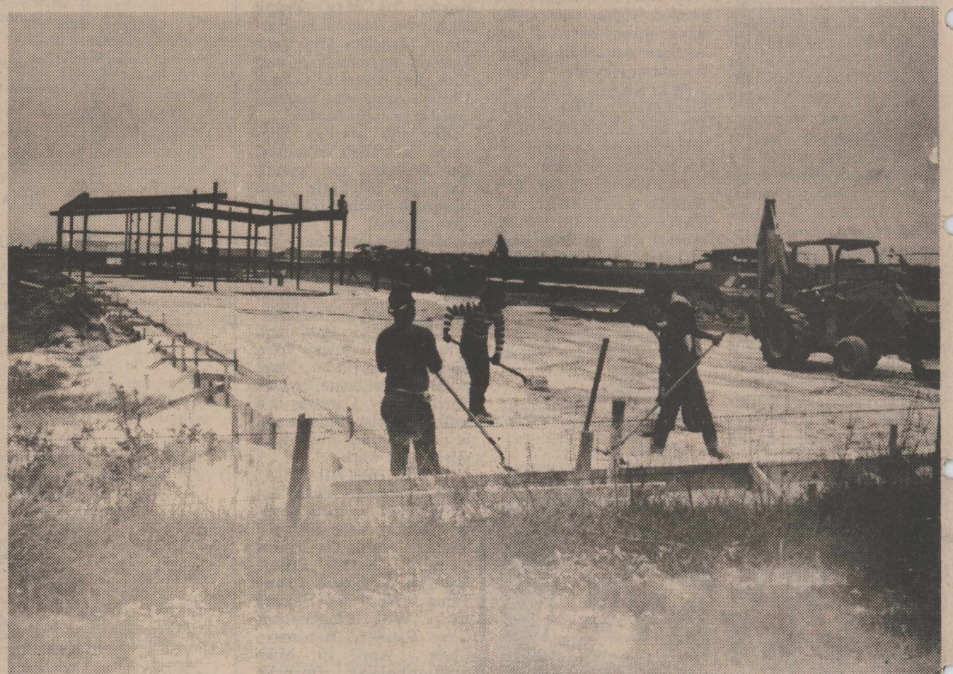
Hangars are going up at the airport
