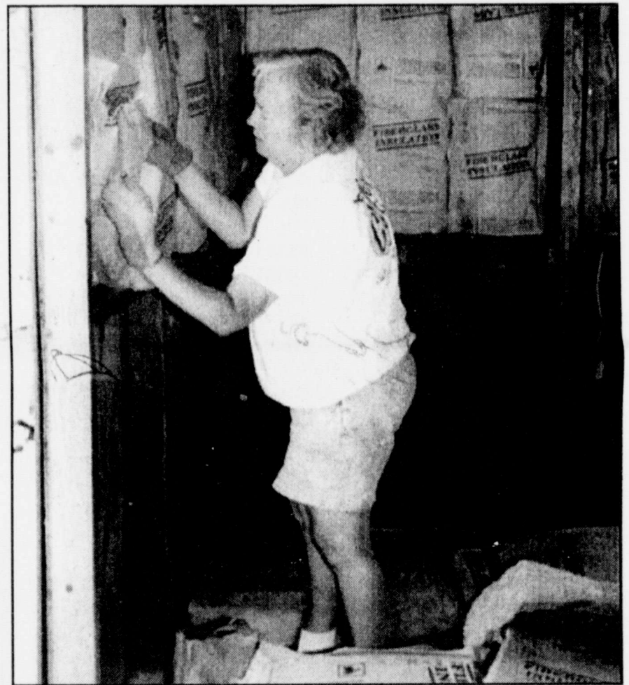
JANE BOURDO makes quick work of cutting and installing insulation.
