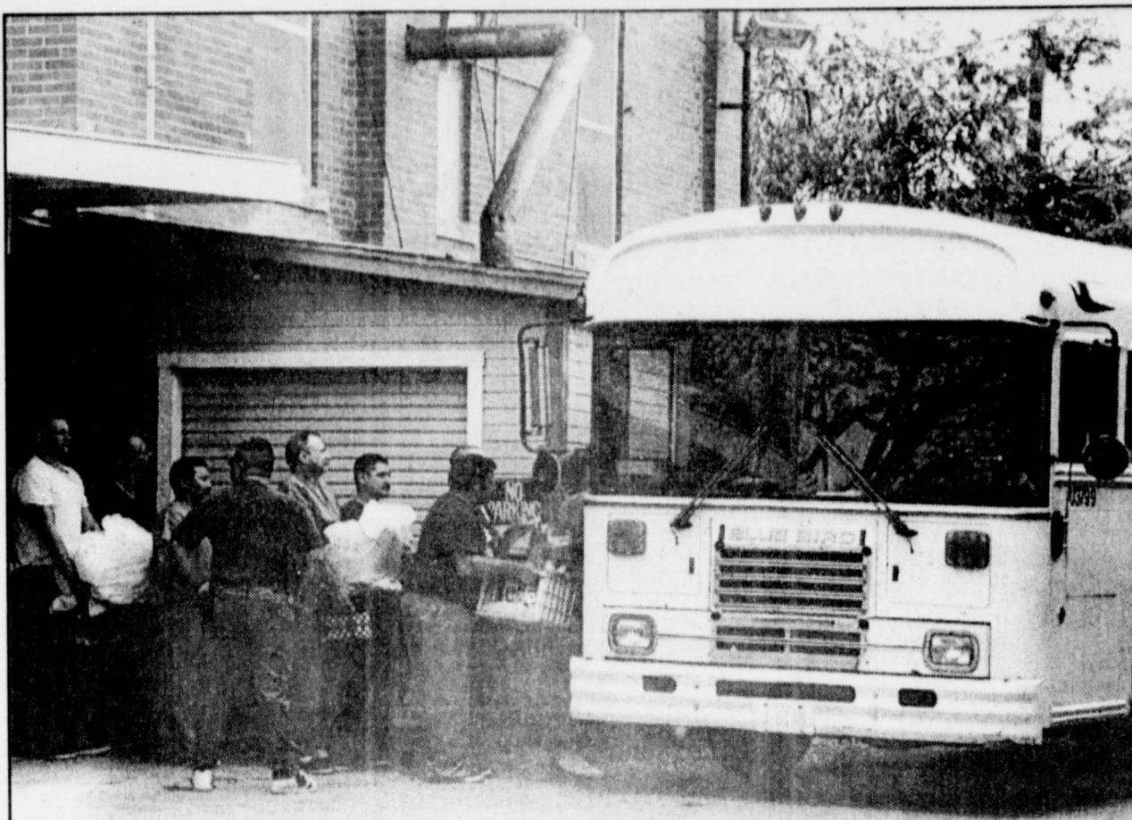
INMATES IN THE RUNNELS COUNTY JAIL were moved to the new jail facility on Saturday, April 10. With the assistance of a U.S. Border Patrol bus, all 30 inmates and their personal belongings were moved in one trip. Runnels County Sheriff Bill Baird supervised the move with the help of deputies, Ballinger Police Department, Winters Police Department, Game Warden Lane Pinckney and Texas DPS troopers.
