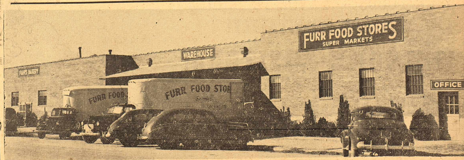
General office and warehouse, which houses the Furr creamery and bakery, is located at Lubbock, Texas, and is shown above. Here big Furr trucks roll out daily to all points with super market merchandise.
