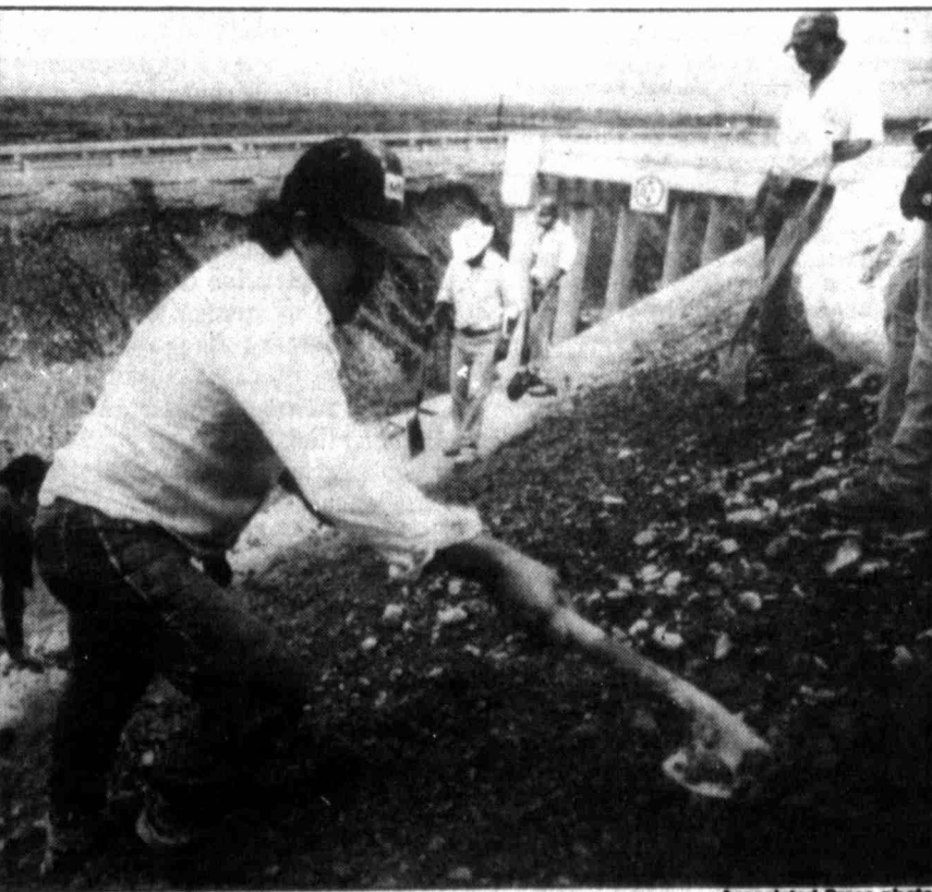
Workers in Monterrey, Mexico, perform maintenance on the new Cadereyta-Reynosa toll highway in late July. It runs from the northern Mexico industrial city of Monterrey to the United States border. Northern Mexico is preparing for increased trade with United States with or without free trade agreement.
