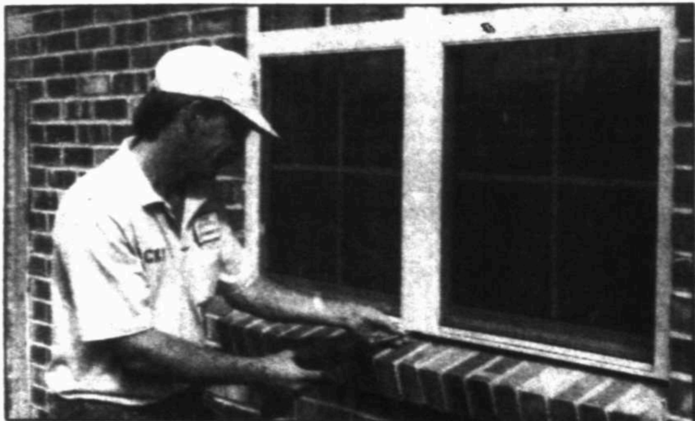
Mid-West Door & Window technician Rocky Pease installs an energy-efficient replacement window in a Midland home. Call 682-4632 for a free estimate.
