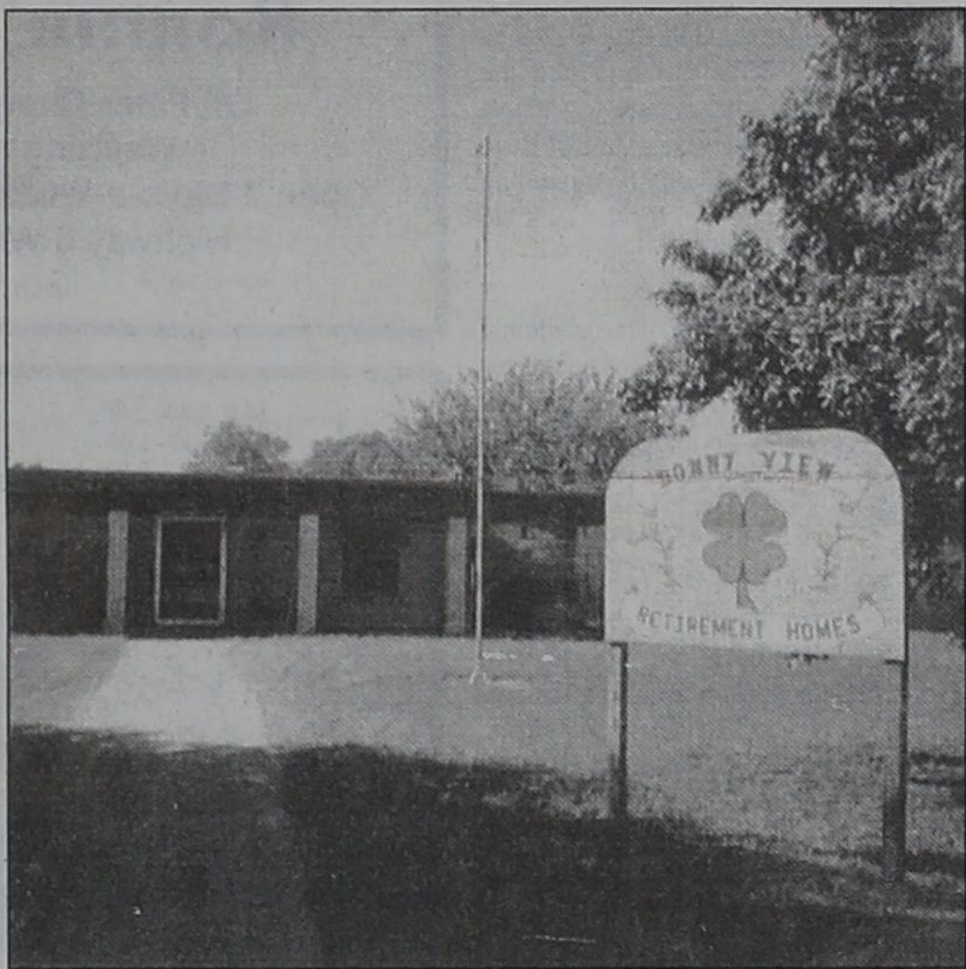
Bonny View Retirement Home in Gorman, Texas (the late Blackwell Hospital) located at 430 W. Roosevelt, and owned by Paul and Bonnie Williams of Carbon, Texas.
