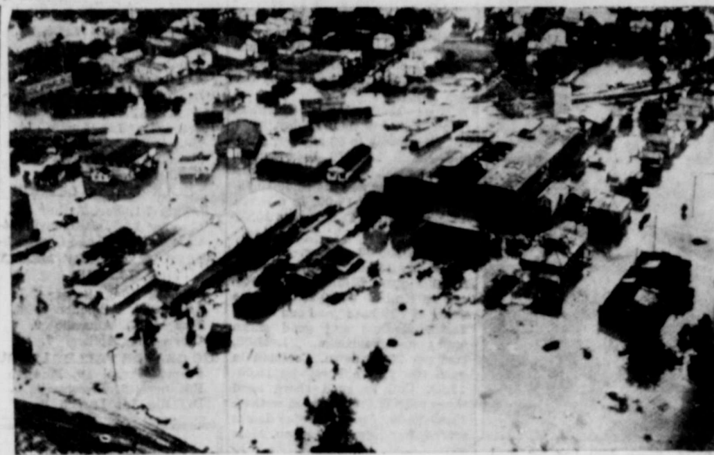
THOUSANDS FLEE OHIO FLOOD—Aerial photo shows portion of Crooksville, O., inundated when a four-hour cloudburst left a 25-square-mile area in southern Ohio almost completely flooded. Thousands of residents in the rich pottery-making and coal mining district were forced to flee their homes before the rising waters. (NEA Telephoto).
