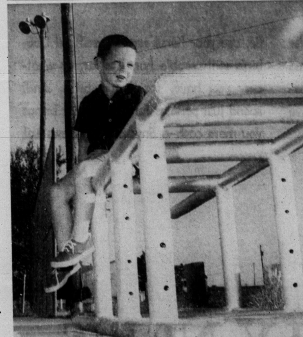
A STAND IN TIME—Erecting of permanent-type judging stands for the Towle Park tennis courts is being accomplished by park superintendent Russell Jones, and they will be available for use during the Scurry County Tennis Tournament — open to all current Scurry County residents — which will begin tomorrow. Here, Eddie Wheeler (son of Mr. and Mrs. Garland Wheeler) checks out one of the three standards which are to be set on end and mounted in concrete today. (Photo by Jackson)
