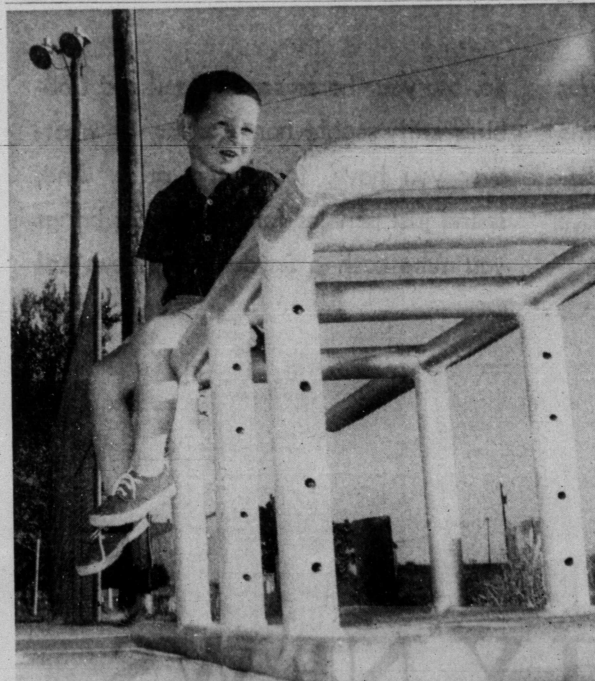
A STAND IN TIME—Erecting of permanent-type judging stands for the Towle Park tennis courts is being accomplished by park superintendent Russell Jones, and they will be available for use during the Scurry County Tennis Tournament — open to all current Scurry County residents — which will begin tomorrow. Here, Eddie Wheeler (son of Mr. and Mrs. Garland Wheeler) checks out one of the three standards which are to be set on end and mounted in concrete today. (Photo by Jackson)
