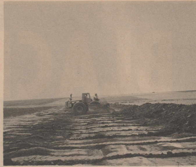
GRASSED WATER WAY just completed on the W. T. Hall Jr. and John Speck Jr. farms. Both farmers are members of the Lamb County Soil and Water Conservation District.
