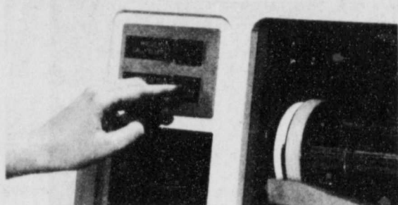
C Close the cap and the carrier locks itself. Nothing can slip out in transit. Place the carrier in the tray and press the button marked, "press to send carrier".
