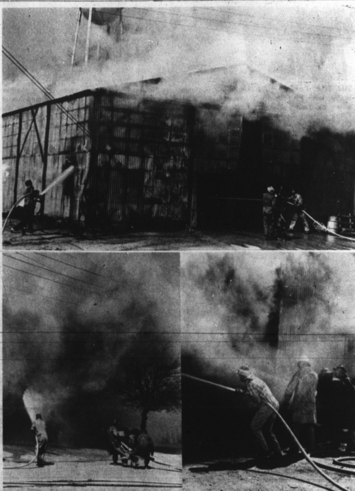
CITY BARN BURNS — Smoke was dense and heat intense as firemen arrived at the City Barn on New York St. Thursday afternoon. The building, which served as maintenance garage for city-owned equipment, was destroyed by the blaze. (Staff Photos by Wain Miller)
