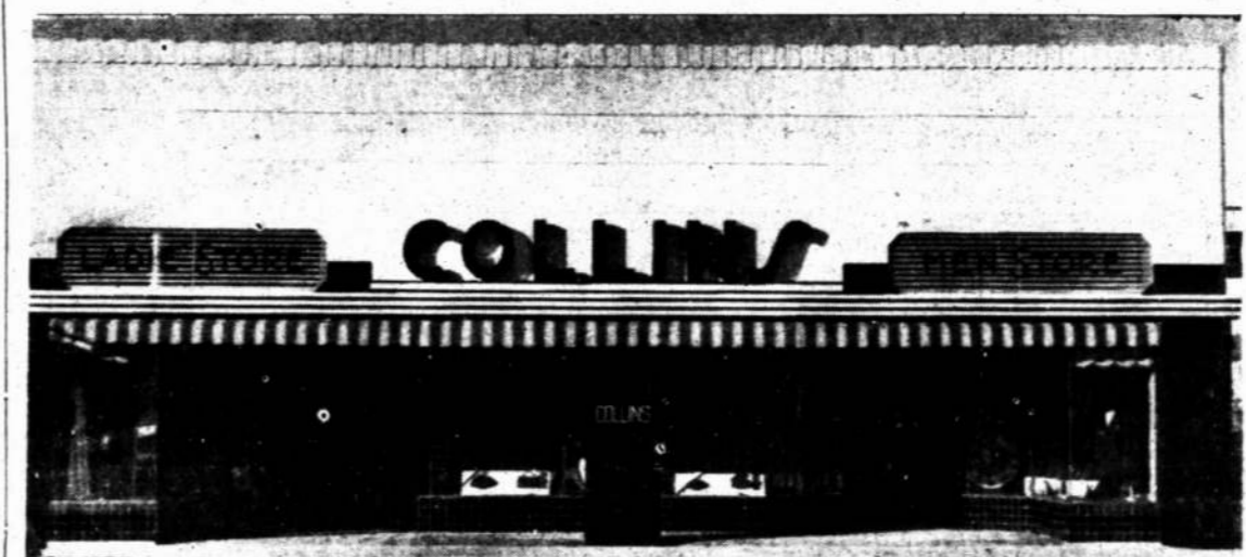
Above is pictured the newly remodeled Collins Store in Lamesa. This new front is of white stucco and black construction tile. It is modern in every respect, and the most modernistic lines have been followed throughout. The large display windows may be seen in the background. This is now one of the most modern store fronts to be found in West Texas, and is another step by this progressive firm in keeping pace with the growth and development of Lamesa and surrounding territory.
