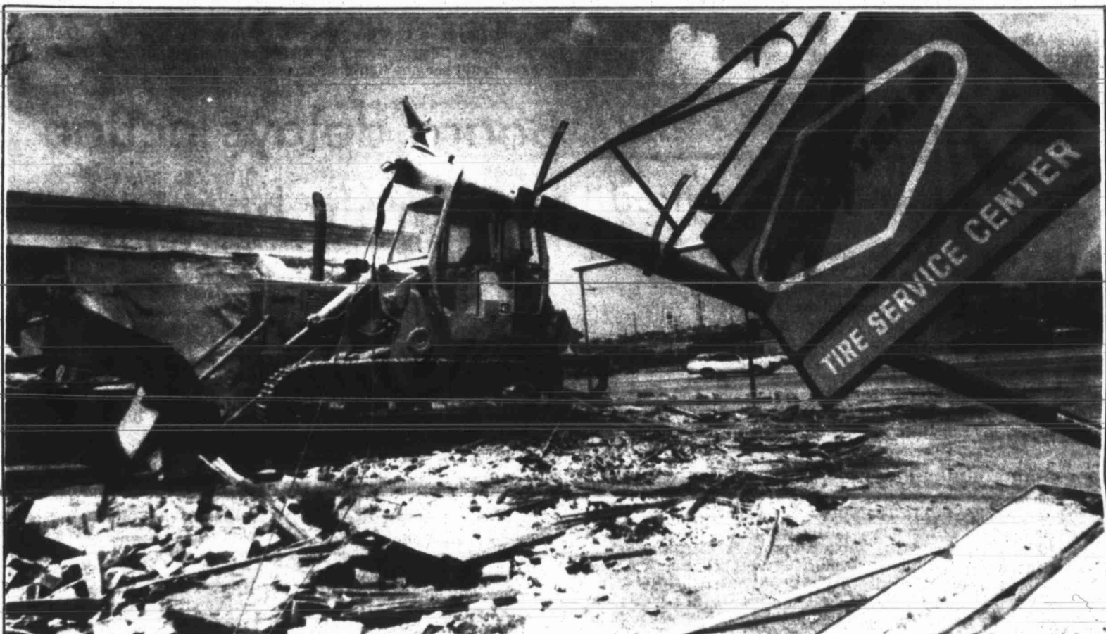
A bulldozer destroys a vacant gasoline station to make room for a convenience store being built by a San Angelo development company.
