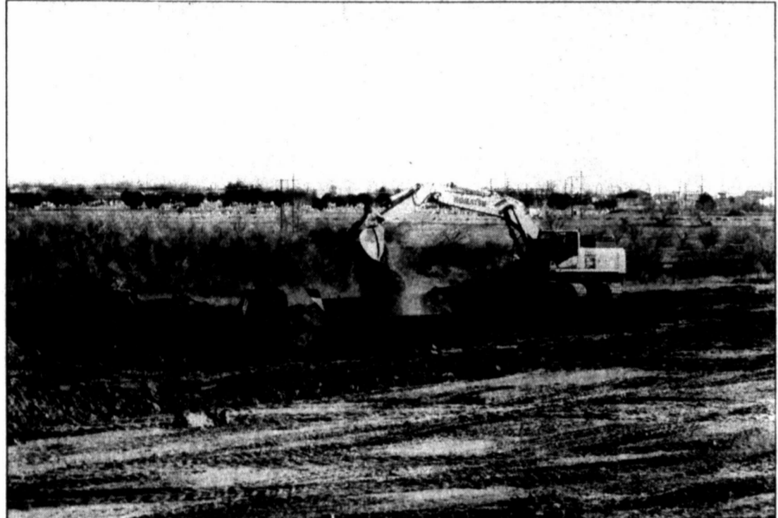
MAKING HAY WHILE THE SUN SHINES - Dirt workers have been building up the soil for a foundation for the new Colorado ISD K-8 campus. The foundation of the school must be built up eight feet to be in compliance with the 100-year flood plan.
