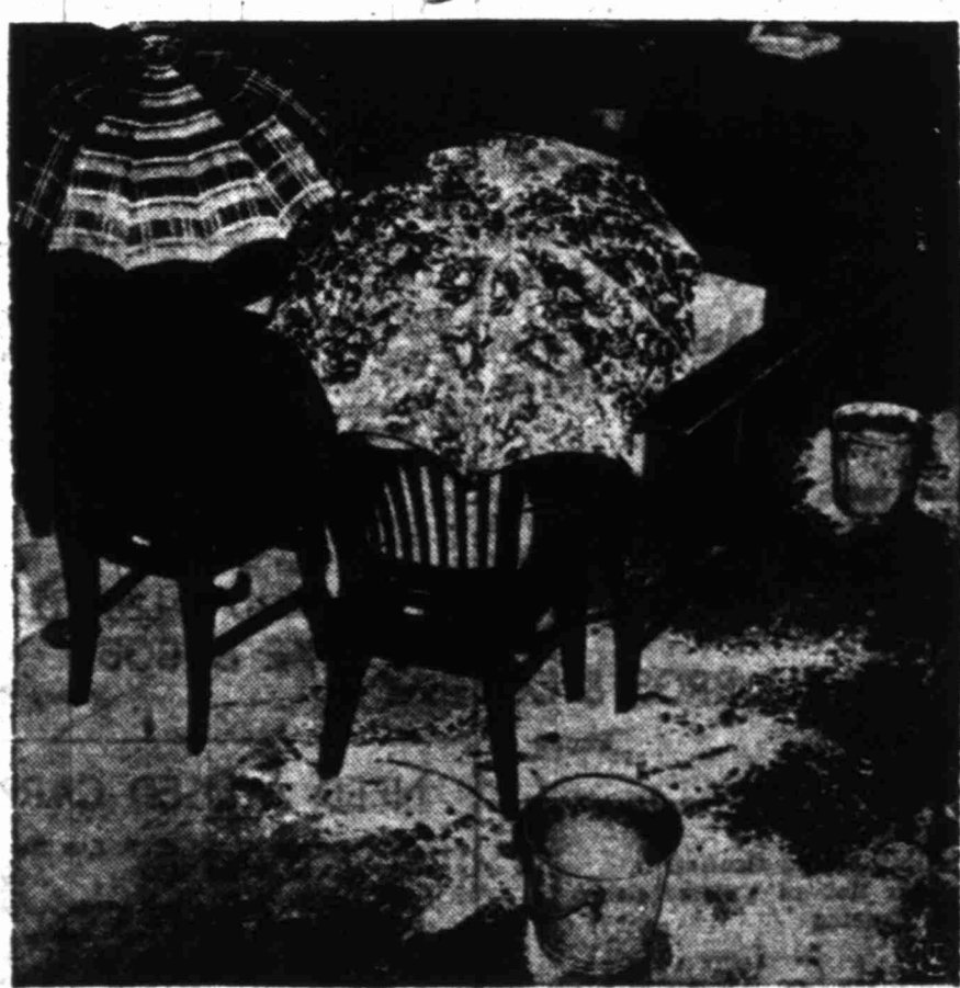
Clerks in the Internal Revenue Department in Chicago work under cover. Umbrella cover, that is. The U. S. Court House, where they work on the second floor, leaks, and umbrellas and buckets are needed to catch the drops.
