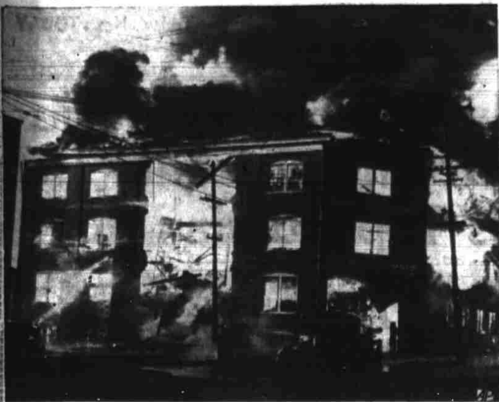
LUMBER YARD BURNS—Fire destroyed the large yard of Wilmington (Del.) Sash and Door Co. and eight adjoining houses. This picture was taken shortly after part of one side of the main building collapsed, showing the entire interior of the building on fire. (AP Wirephoto)
