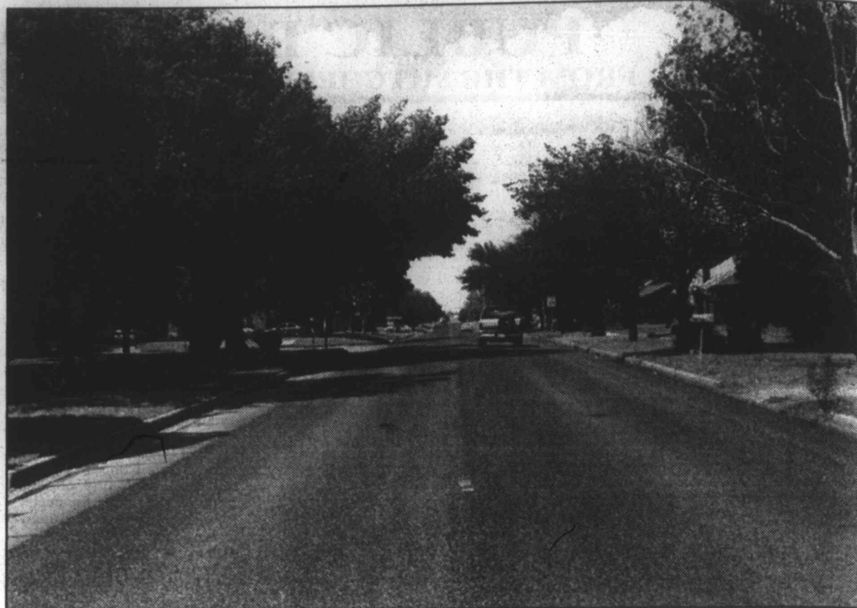
HICKORY STREET repaving from Interstate 20 to East Second Street was temporarily suspended by Price Construction Co. of Big Spring, but plans are for the final coat to start being laid on Monday. The project should be finished in three to five days, a highway department official said.
