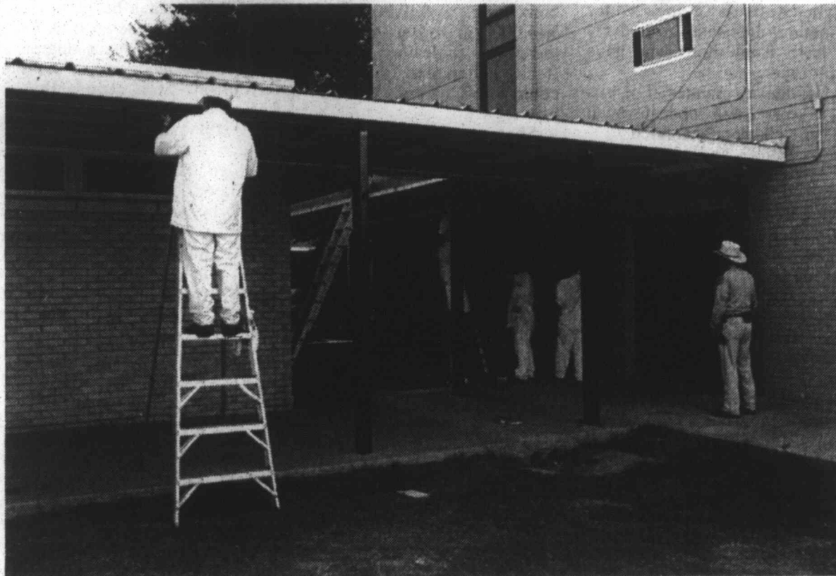
BACK TO SCHOOL painting was underway at Colorado Middle School by a crew of Wallace Unit inmates. Students will return to school here on Thursday, Aug. 13, and in Loraine and Westbrook on Aug. 12.
