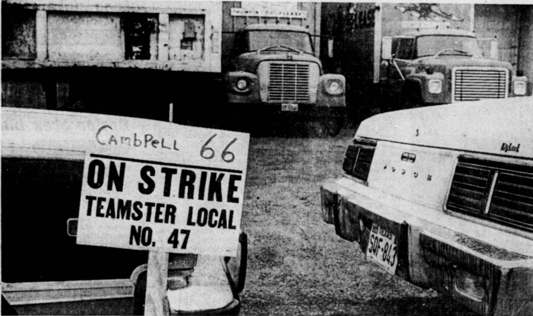
TEAMSTERS HAVE SIGNS OUT, BUT NO PICKETS AT THIS SITE TODAY ...at Campbell 66 Express truck terminal in Wichita Falls (Photo by Jim Cochran)
