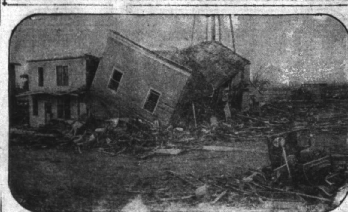
The Federal women's club at Rockford, Ill., is pictured above. Heavy winds were blowing in the Rockford storm, and the property damage ran into millions. Brick walls were blown in like eggshells in the wind's fury. It was in the factory that most of the deaths occurred.
