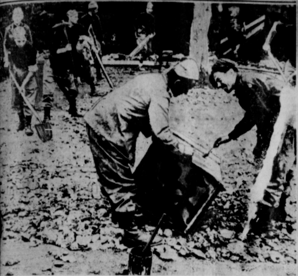
An army isn't going to get into a rut in the impending war with Ethiopia if forehanded preparation is made. These blackshirt troops on the Eritrea front in Africa, are building hard roads over move supplies across heretofore trackless terrain. Those in the foreground are camouflaging a machine gun.
