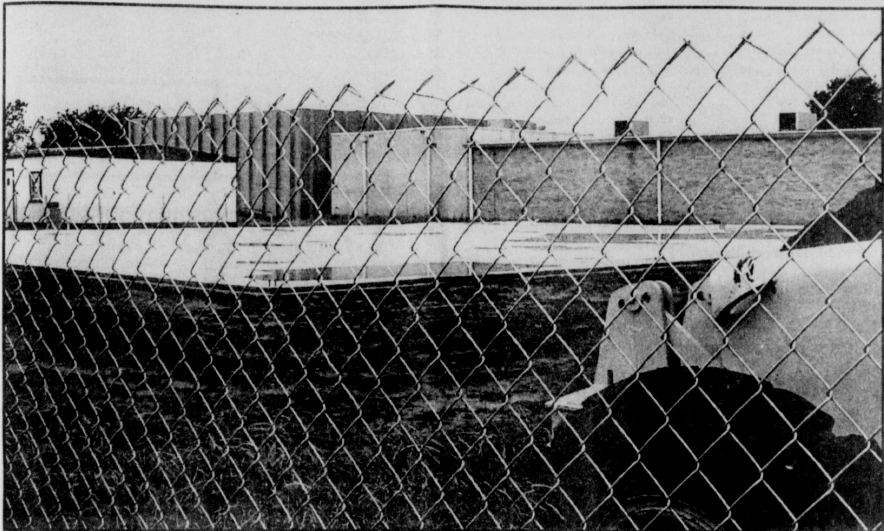
PART OF THE EXPANSION underway at Bradford Elementary includes classrooms on the East side of the building. Other
