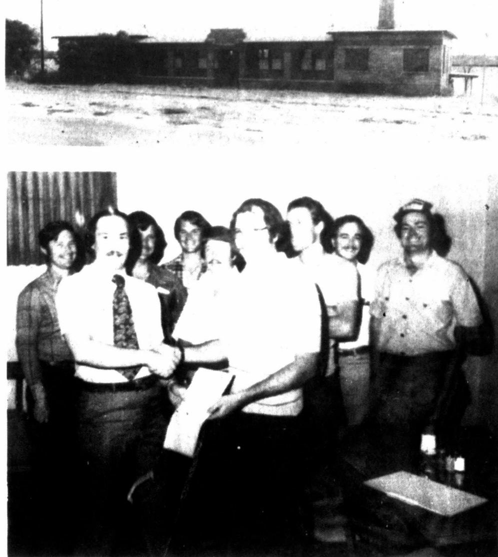
COLORADO CITY JAYCEES and the Mitchell County Boys' Club have joined forces to renovate the former American Legion Building at 3rd & Chestnut. The building has been used by the Boys' Club for a number of years but they needed help and the Jaycees needed a building to help carry out their projects so an agreement was reached. In picture above, Jaycees' President Dr. Don Bennett, right, and Boys' Club President Pat Barber, left, are shown with members of the Jaycees after both organizations approved a contract on their agreement Wednesday.
