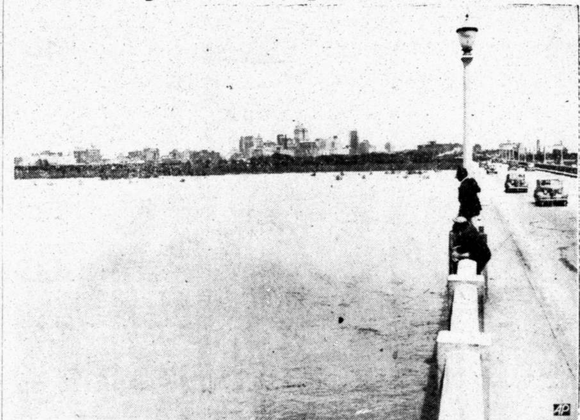
Swollen by flood waters, the Trinity River at Dallas normally a tiny stream, crested at 45.43 feet, highest since the historic flood of 1908 when it surged to 52.6. This view shows the Dallas skyline in the background and the Corinth Street viaduct at the right.
