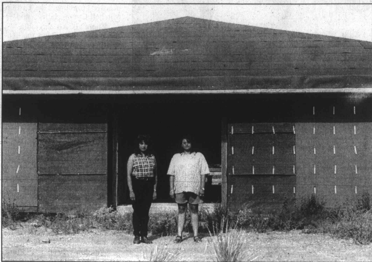
BETTY CASAREZ, left, director of New Discovery Child Care Center, and her assistant, Melissa Lara, will move the center into this new day care building that is being constructed in the 1100 block of East Ninth Street.
