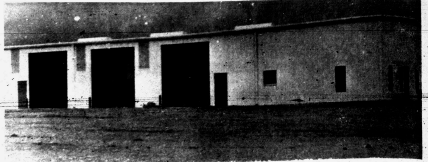
CRC WIRELINE - CRC Wireline, presently located north of Snyder on the Clairmont Highway, is having new quarters constructed off the Lamesa Highway west of town, approximately a quarter-mile north of the Ponderosa Motel. The new facility, shown above, measures about 50X100 feet and replaces the existing 38X75 building. The new building is expected to be moved into in about two to three more weeks. (SDN Staff Photo)
