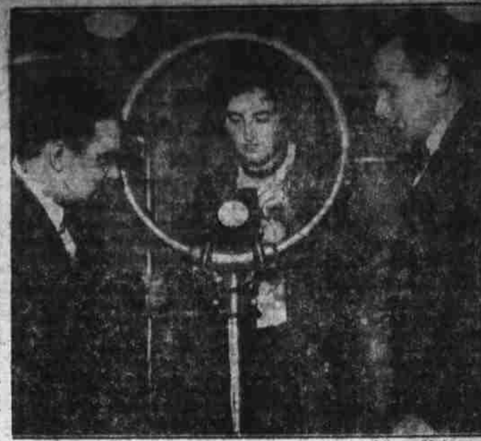
Jimmie James (left), pilot, Alma Griffin and Gerhard Fisher aboard a plane over Los Angeles, test a new radio direction finder by which a pilot can tune in on a radio station and be guided to it by the finder indicator. The device was designed by Fisher and perfected by Herbert Hoover, Jr.
