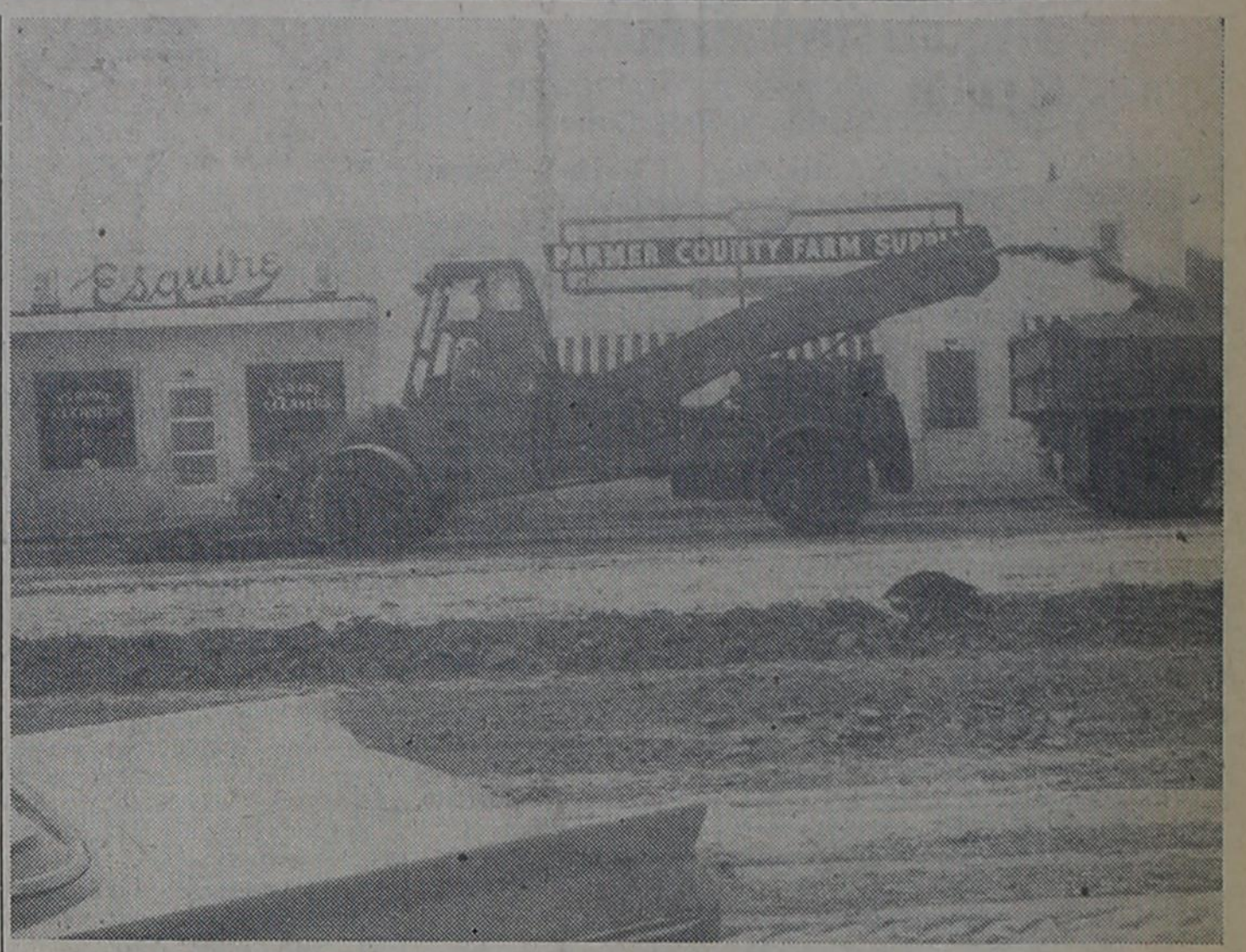
SIGN OF PROGRESS—This street equipment is a sign of the times in Bovina as Main Street is being prepared for paving. A brand new city-fied type street is to be the scene in Bovina after the construction is finished.
