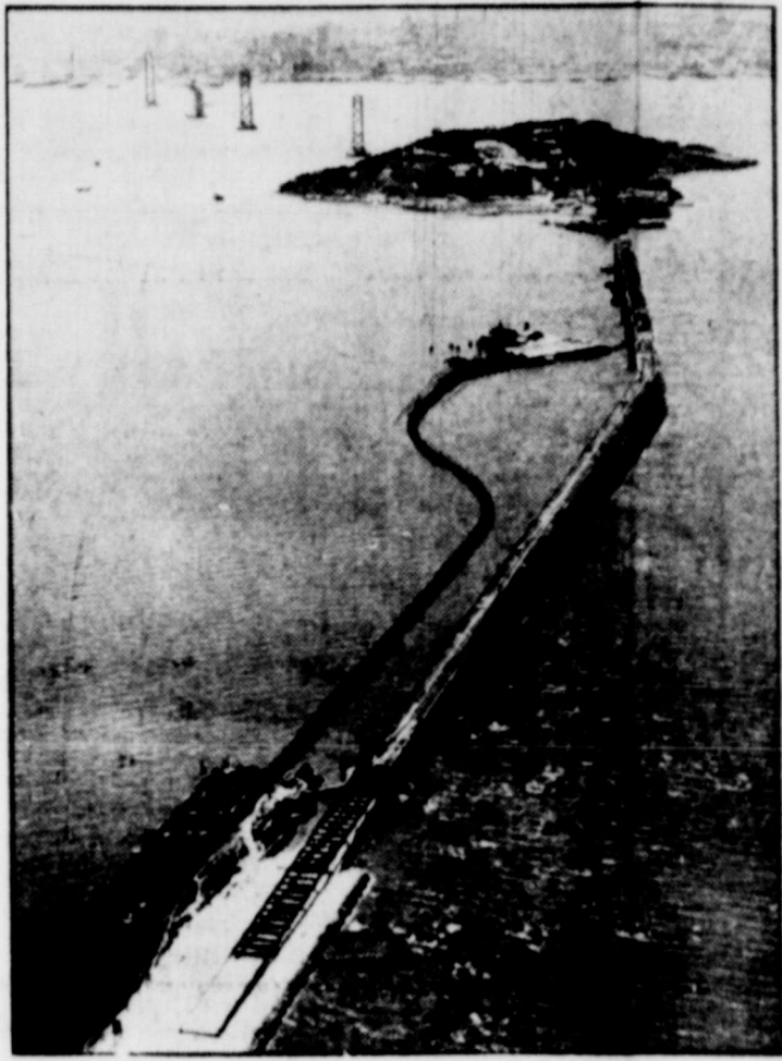
The San Francisco-Oakland bridge is rapidly assuming a definite shape and becoming a concrete example of great engineering achievement. The above view, taken from the air above Oakland, Calif., shows the eastern span reaching toward Yerba Buena Island, center anchorage of the bridge. Beyond the island may be seen the towers which will support the western span of this great bridge, joining the two shores of San Francisco Bay.
