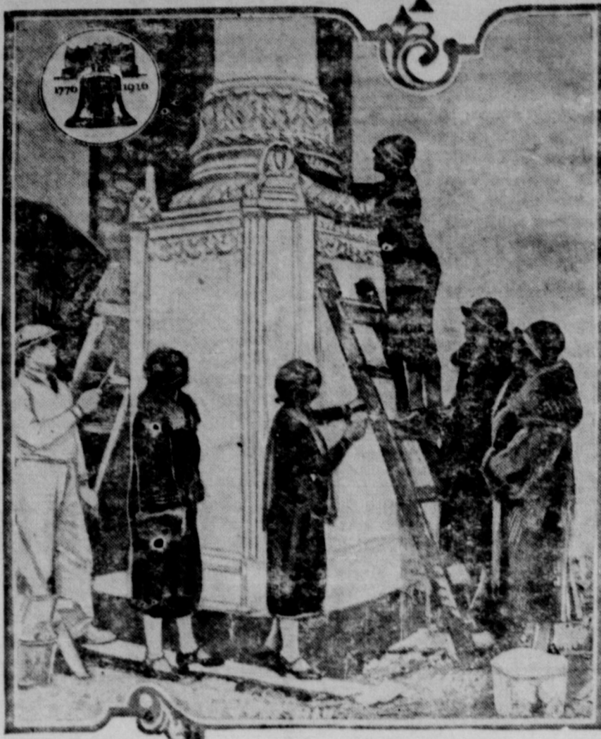
Young women artists turn from their jars of color and paint brushes to assist plasterers in setting ornaments in place atop huge pylons which adorn the main entrances to the Palace of Agriculture and Food Products, of the vast exhibition buildings which forms a part of the great Sesqui-Centennial International Exposition being staged in Philadelphia from June 1 to December 1 to celebrate the 150th anniversary of the signing of the Declaration of Independence. Climbing ladders and walking along rickety scaffolds is nothing new to these young ladies, but each time they do it they get a thrill.
