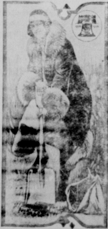
Under this young woman's skillful hands the front of the Administration Building of the Sesqui-Centennial International Exposition Association quickly takes on a delightful aspect. She directs gardeners where to place the small trees and shrubs about the great stucco building. She is doing her share to make the big celebration of the 150th anniversary of the signing of the Declaration of Independence a success.
