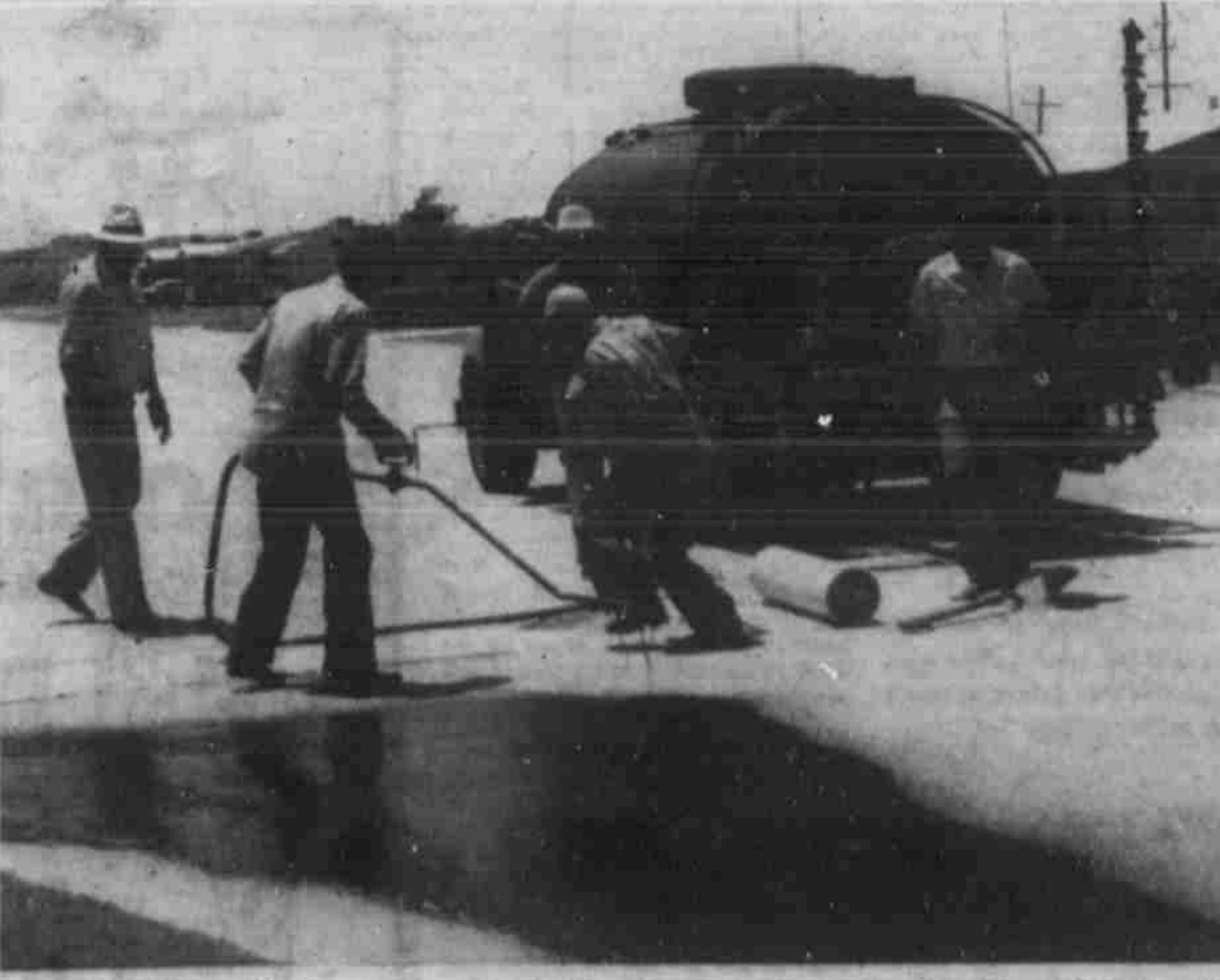
EVERYBODY'S BUSY —The above activity, being repeated many times daily here, took place at the corner of Avenue Q and Seventh Street during seal-coating of Seventh. The surfacing machine in the background has just put one streak of asphalt on the street and workmen are rolling paper to assure a straight edge at where the surfacing stops. At the extreme left is Bob Isbell, engineer for the City of Post and at the extreme right is R. L. Chastain, an official of the C&C Asphalt Paving Co., contractors on the re-surfacing project.—(Staff Photo).
