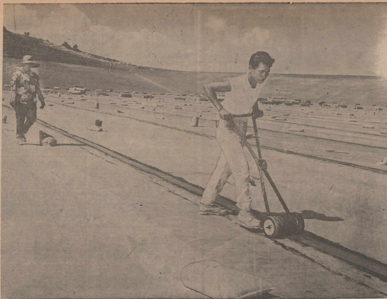
ROLLING AND SEALING a seam lap is final operation on rubber lining for Hawaii's Kualapuu Reservoir, largest rain-harvesting reservoir of its kind in the world. Its purpose is to divert misguided rainfall in Molokai which falls mainly on the wrong side of the mountains, seldom on the plains where it's needed.
