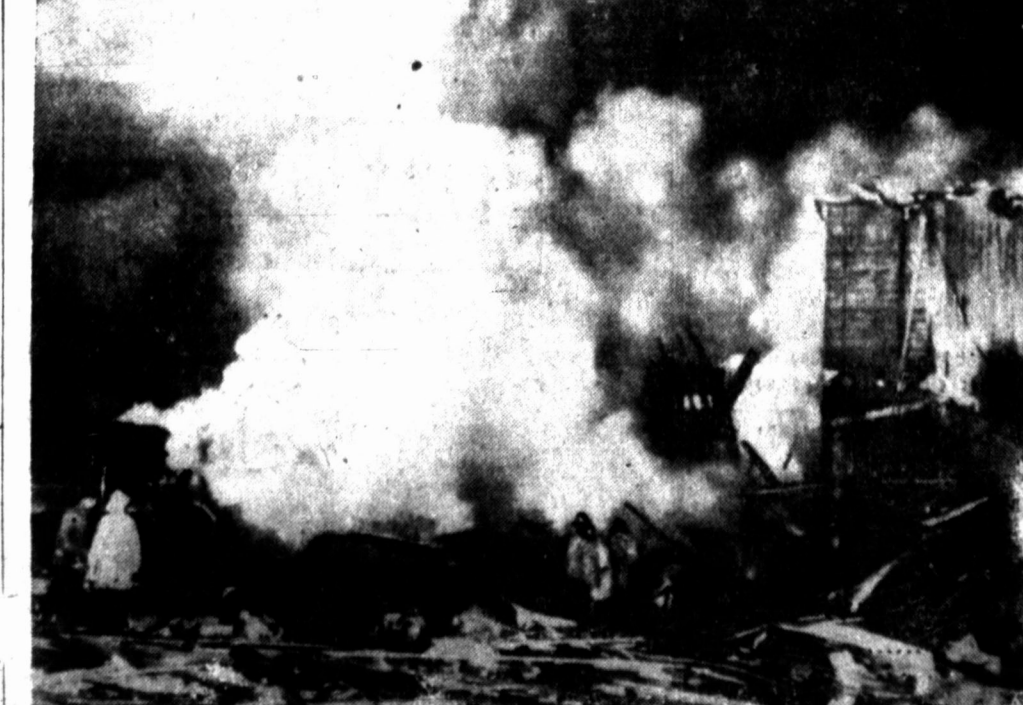
EXPLOSION DESTROYS OFFICE BUILDING—Firemen battle flames in the wreckage of the Postoffice building in Portland, Ore., after leaking gas blew up the structure. Only one person, an engineer who turned on a light that set off the blast, was injured.
